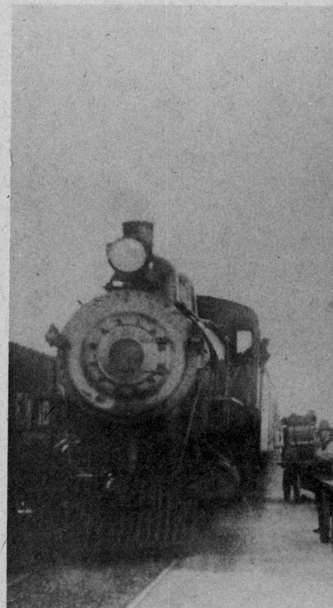
The Fort Worth and Denver City Railroad depot at Memphis, built in 1891, was
