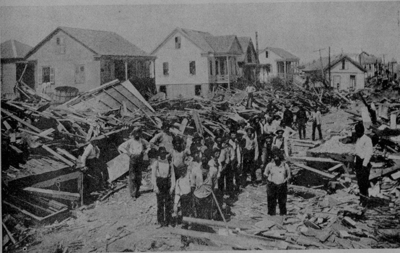
Volunteers removing debris on 21st Street looking south.
