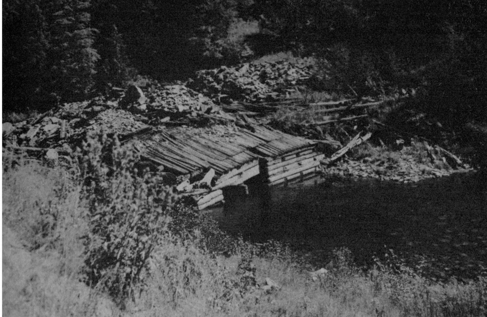
Above, close-up view of the dam on Marble Creek where logs were piled up, then flooded out in high water. Below, remains of the splash dam on Marble Creek. Note the hill in upper right, denuded by the great 1910 fire.
