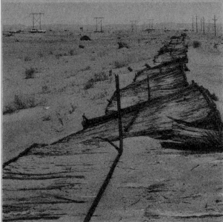
Above, "Old Shaky" was the nickname given this first roadway link between Yuma and Southeastern California, back in 1915. It was constructed of railroad ties laid on top of the sand and locked together with steel bands. As the sand shifted, so did the roadway.
