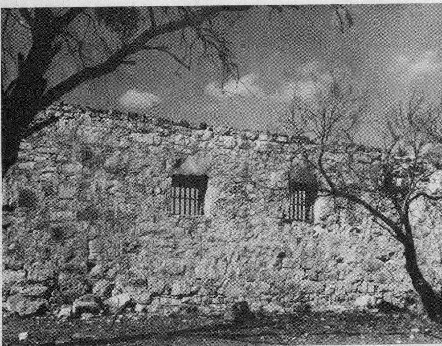
The post guardhouse, located near the middle of Fort McKavett.
