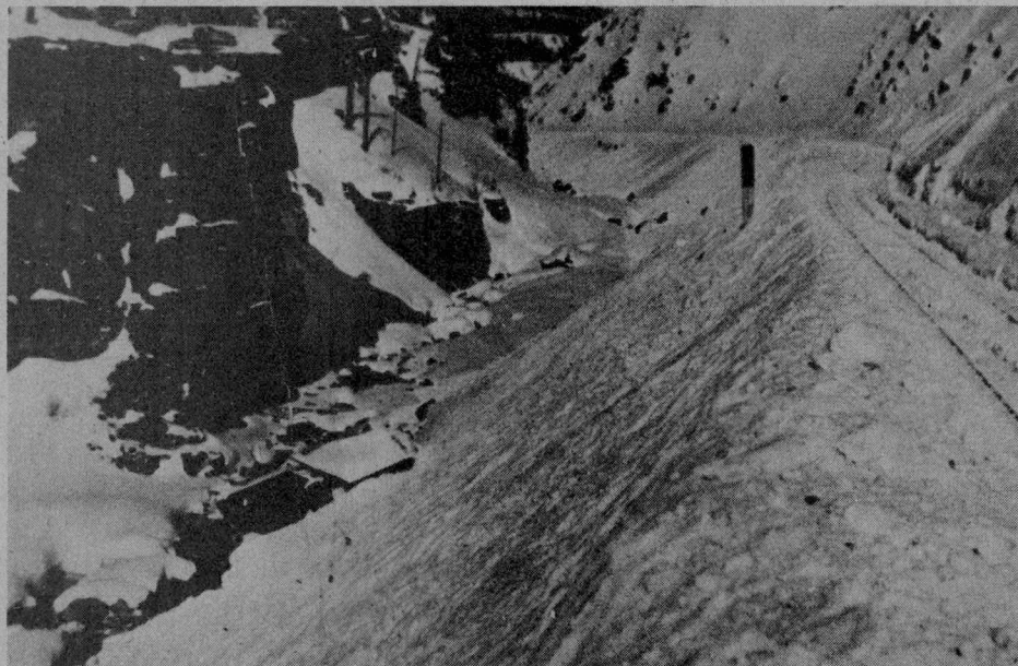
Below. Burns Canyon in 1921, located some three miles north of Rico. Great snow slides were a common problem here, and a rotary plow was used to clear the track.
