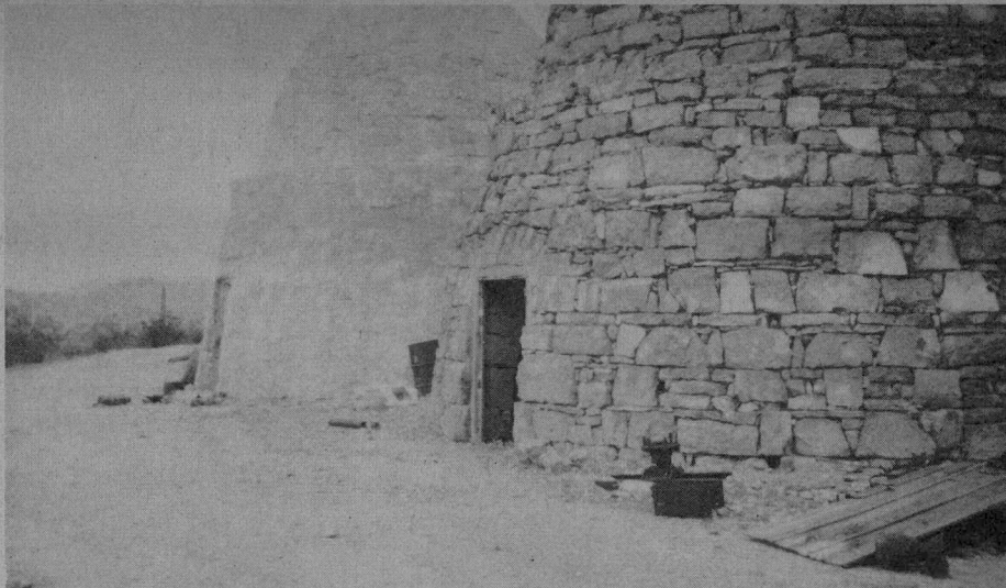
Above, old bee-hive coke ovens. Mining companies made their own coke for smelting ore. These ovens were constructed with stone blocks and no cement. Clay was used for mortar.
