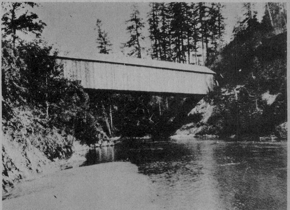
Elwha covered bridge.
