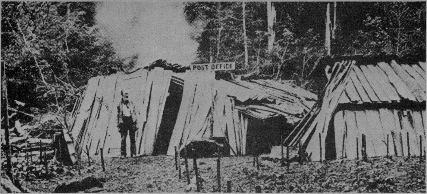
McDonald Post Office, first one built south of Port Angeles, Uncle McDonald, postmaster, standing by. The main room was a hollow cedar stump 143 feet in circumference near the ground. The stump still stands on Mrs. Bertha M. Hartt's ranch, but with its split-shake coverings removed.
