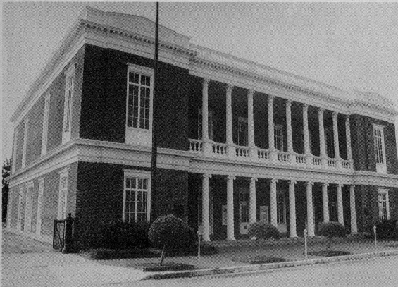
Customhouse in Galveston, Texas. Completed in 1861, it is now a national historic site.
