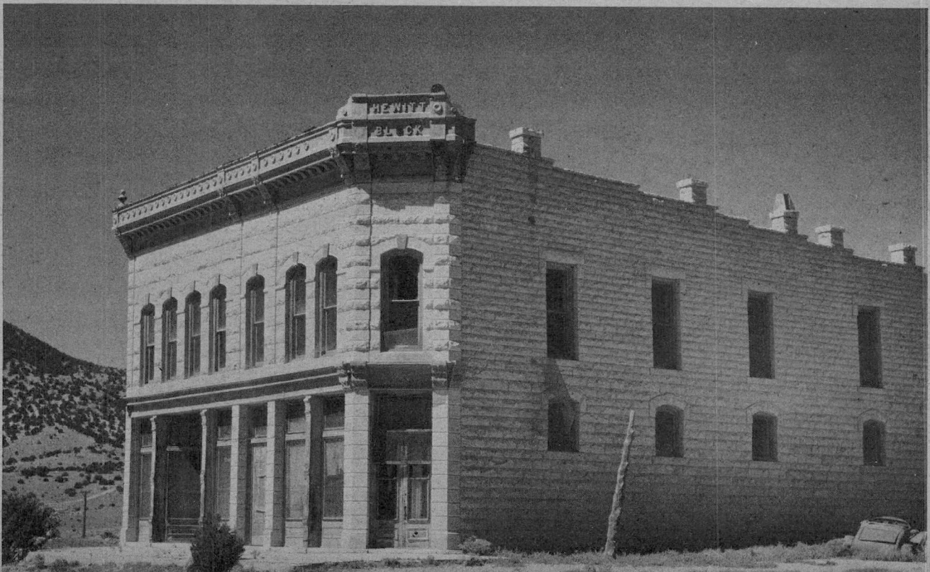
The Hewitt Block, most pretentious business structure in the ghost town of White Oaks, was demolished in October, 1951, for the building material it contained.
