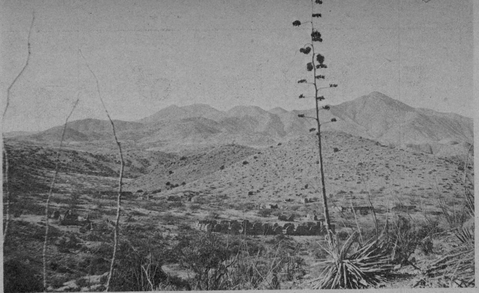
Ruins of old Fort Bowie looking west. The long walls were once the cavalry barracks.
