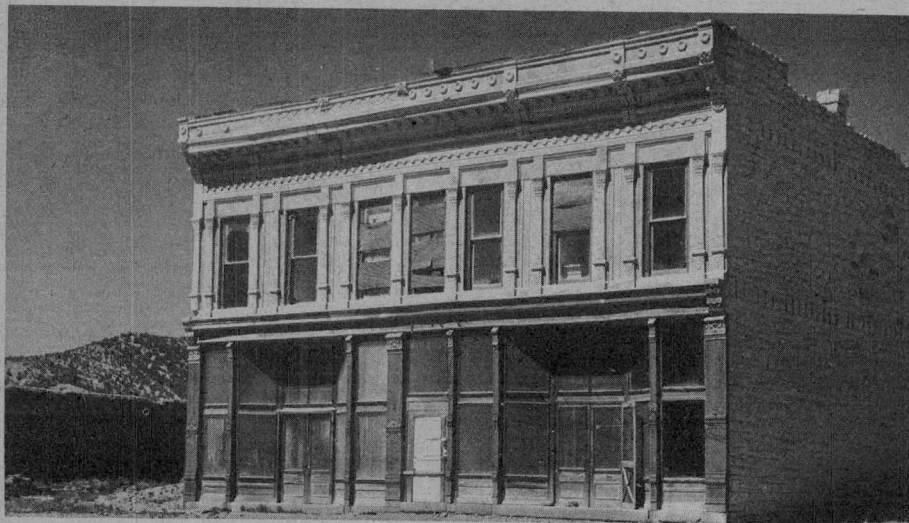
Now vacant, this building formerly housed a general store and post office in White Oaks, with professional offices on the second floor.
