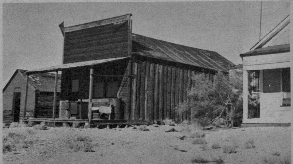
Stores are vacant and grass now grows in once busy Main Street
