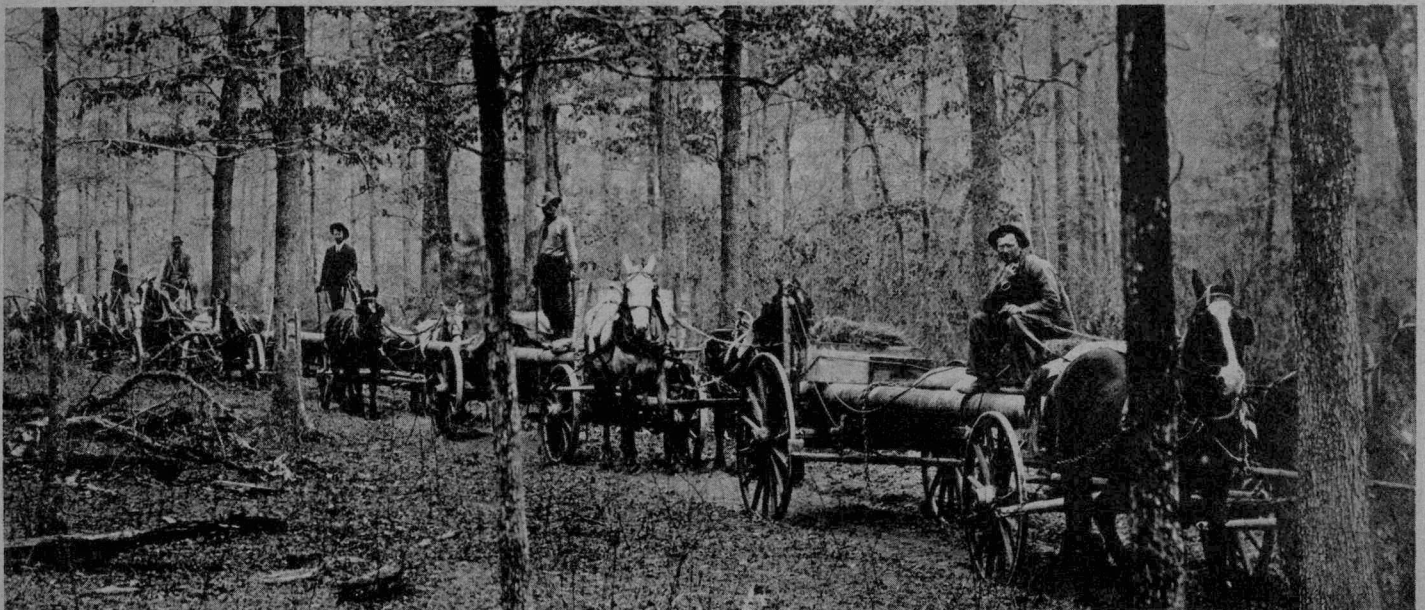
It took a long time to make the trip from Arkansas to Oklahoma with this load of pipe.
