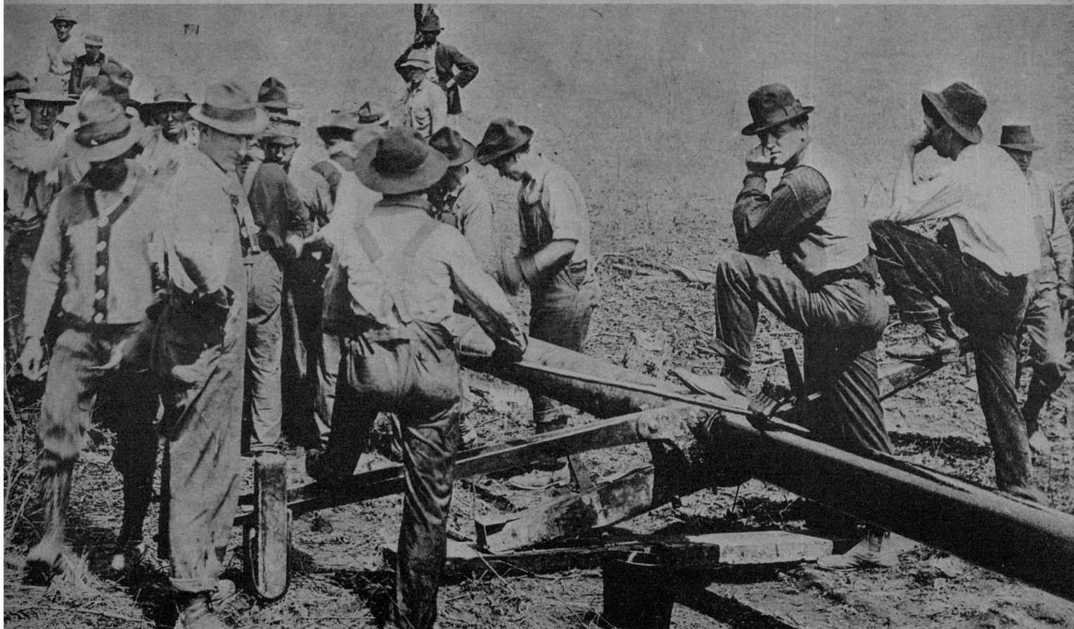
A pipeline crew in the Oklahoma oil fields.
