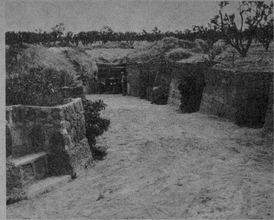
Courtesy Underground Gardens, Fresno, California Entrance ramp to car tunnel
