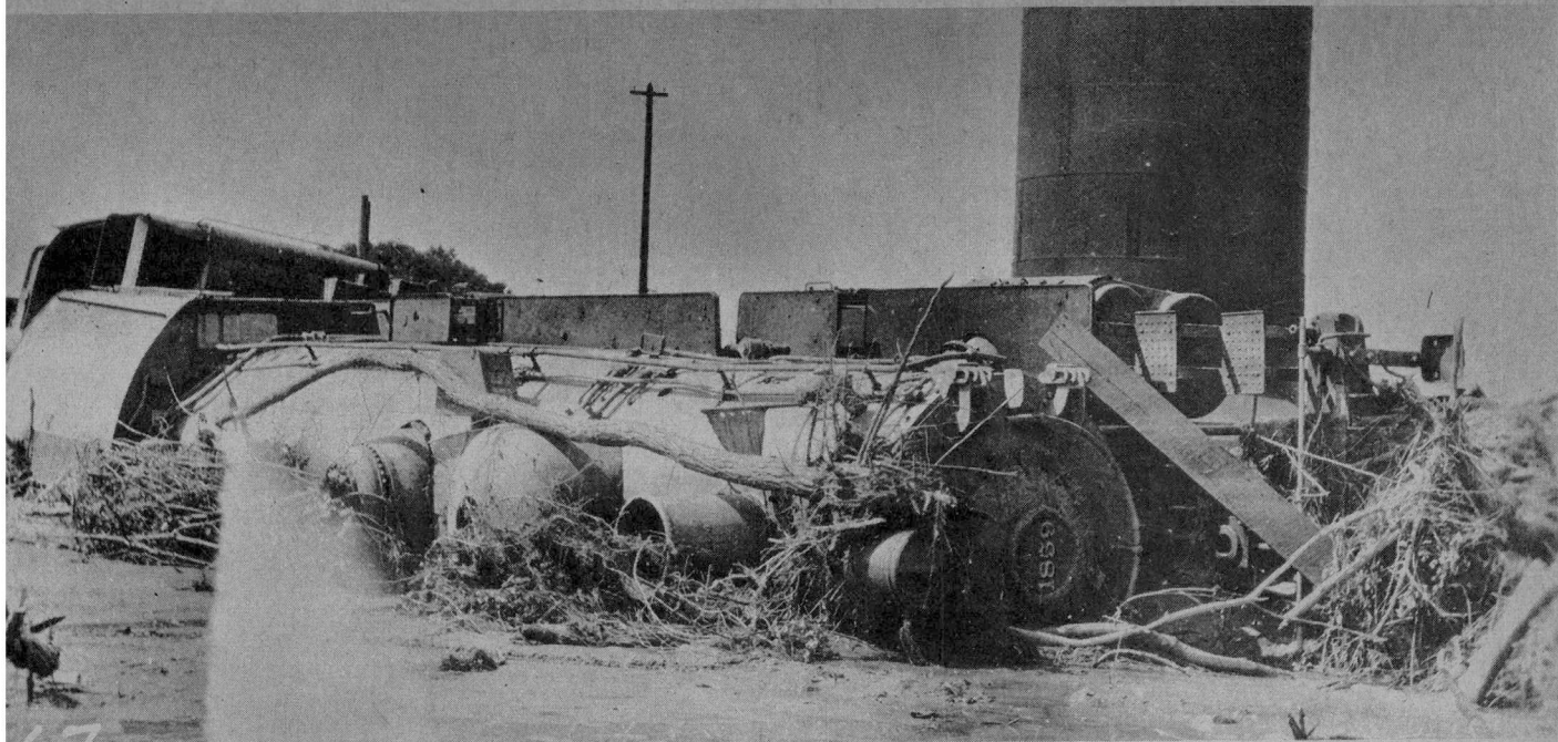
The 1859 on its side at the coal chute.
