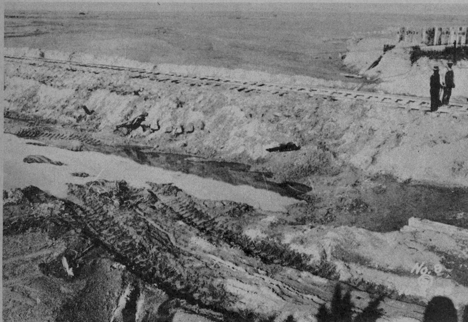
Rio Salado showing the washed-out east approach and channel widening.
