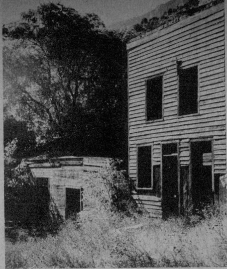
Vacant business building on Main Street, ghosttown of Ophir, Utah.
