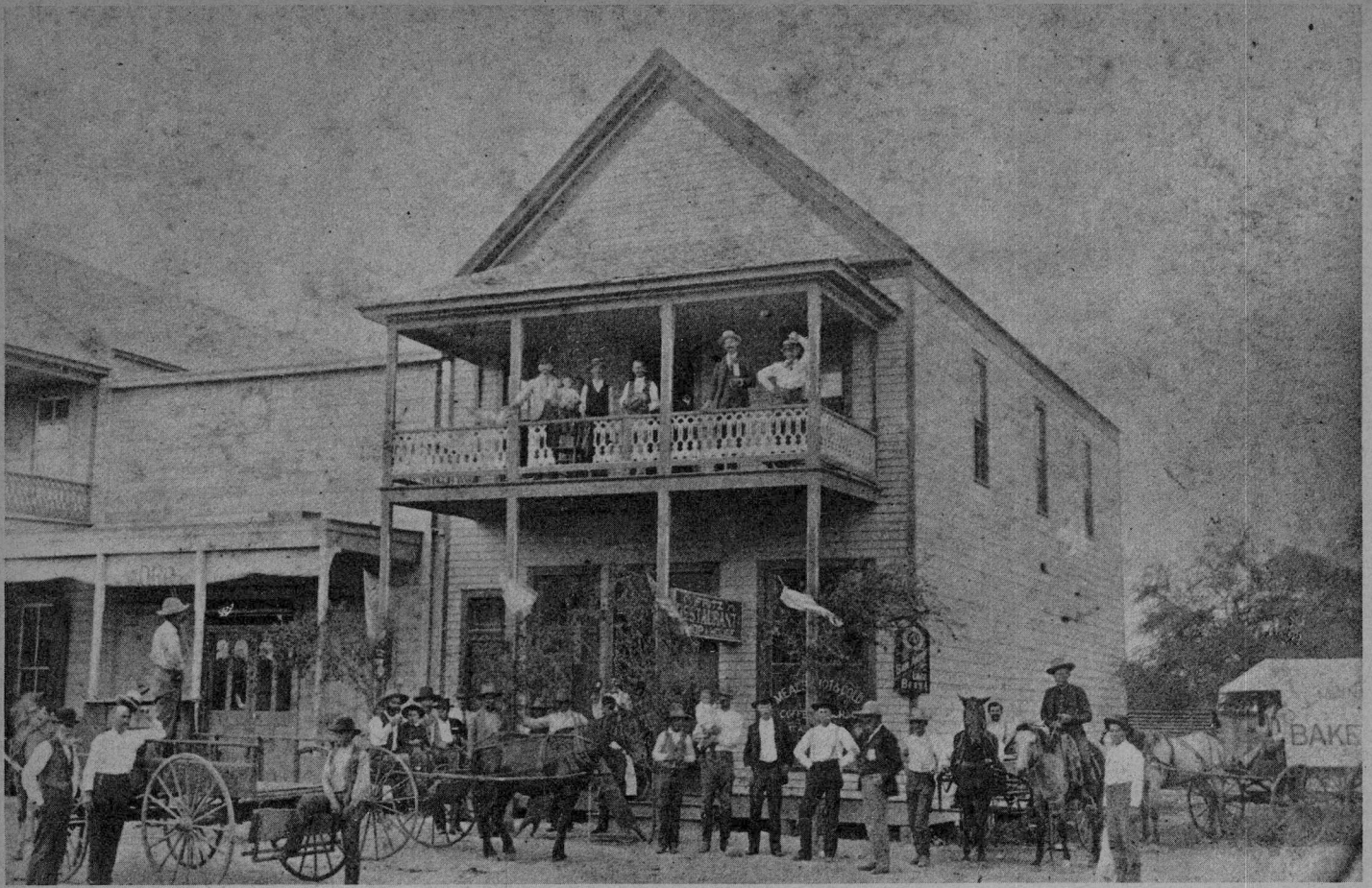
The first business building built in Beeville, Texas. (Grady Harrison, Jr.)
