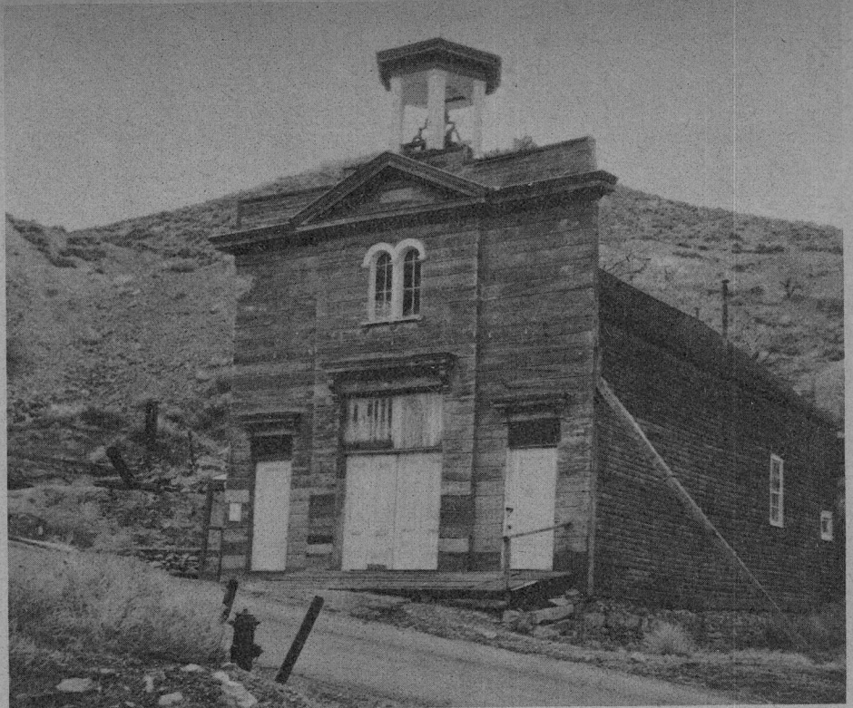
The old fire station in Gold Hill, Nevada. This building has collapsed and been carted away for firewood since the photograph was taken in May, 1948. (Nell Murbarger Photo)
