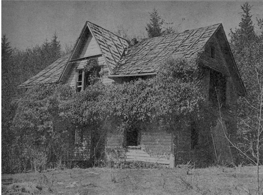
The Nylund home (above) was built in 1905. Mrs. Hilda Nylund Sullivan of Tacoma, Washington, stated that every board and shingle in the house was split and planed by hand. Hemlock trees were squared with a broadax for timber. The second story was built on the ground, then raised into the air and the lower floor built under it. Circular staircases like the one on the right were used in many homes to save space. Below, remnants of old newsprint, dating back to 1894, still cling to the walls of many old homes. A few advertisements (enlarged) give insight into the needs of the day.
