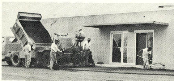
Paving front parking lot.
