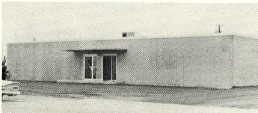
Front on new building under construction.
