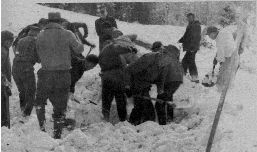
Volunteers dig down to one of the two bulldozers covered by the "Schoolhouse slide." The huge Diesel tractors were desperately needed for rescue work.
