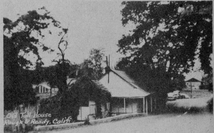
This is Rough-and-Ready's main street today. The old toll house is in the foreground. It was also the Wells-Fargo office and stage depot in the town's old rip-roaring days.
