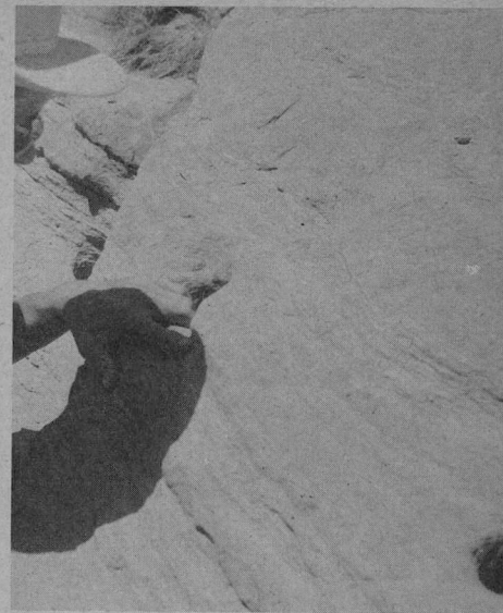
Holes were drilled into the rock for oak pegs which held brush and stone to make a lever roadway over this steep portion.
