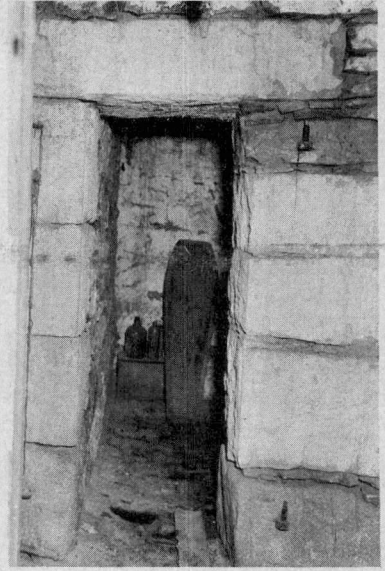
Underground entrance to the dungeon cell. The pins that once held the giant iron doors are seen on either side of the entrance. The room is now used for storage.
