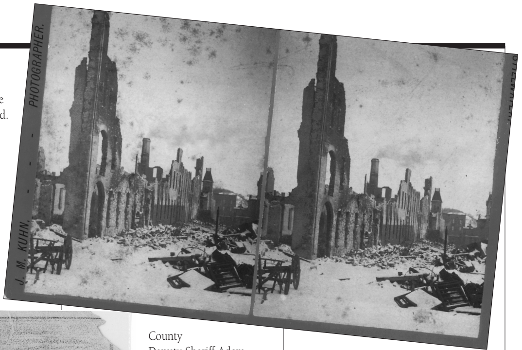
An "inside" view of the damage done to the interior of the prison during the 1884 fire.
