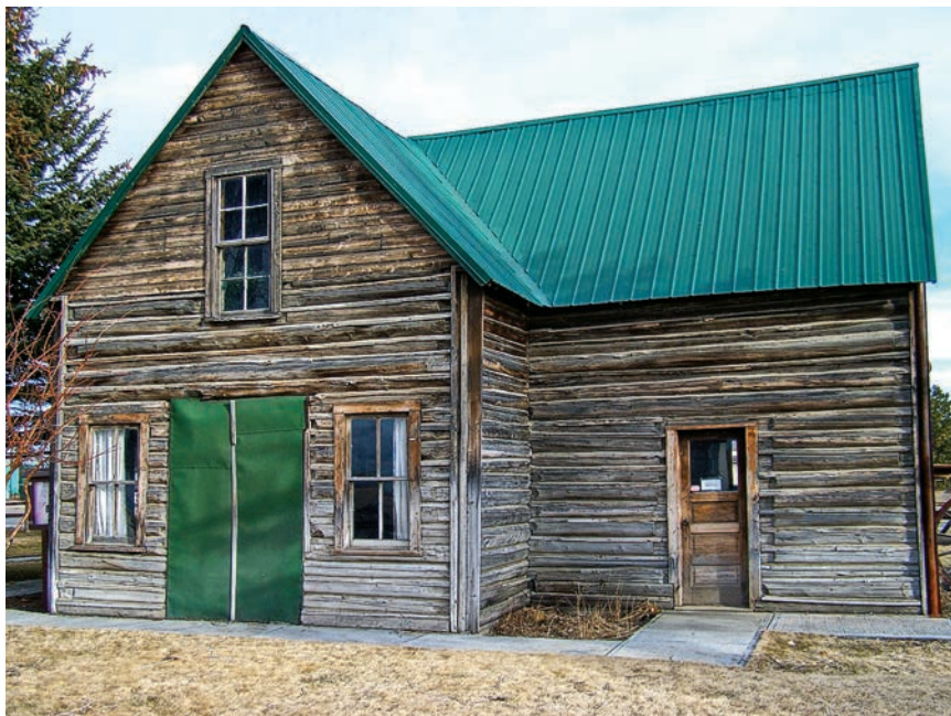
The historic Owen Wister Cabin at the Medicine Bow Museum is currently under major renovations. The author built and lived in the summer hunting cabin in Moose, Wyoming, near Jackson. It was moved adjacent to the Medicine Bow Museum in 1976.
