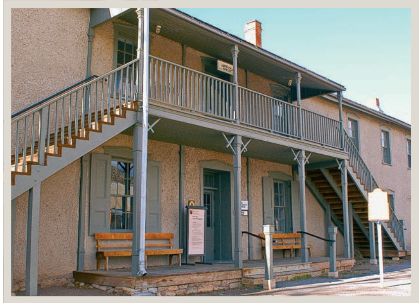
The Lincoln Historic Site includes the infamous courthouse and several other buildings that were actively used during the Lincoln County War.
