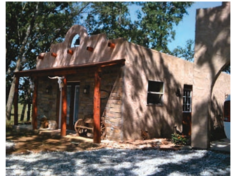
Cedar posts provide stylish support for the porch awning at the Finkenbinder home.
