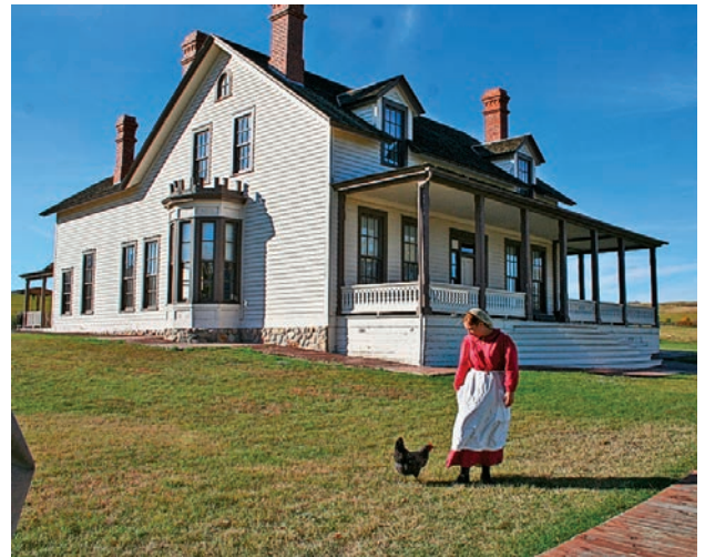
The Custer House is one of the iconic structures restored at Fort Abraham Lincoln near Bismarck, North Dakota.
