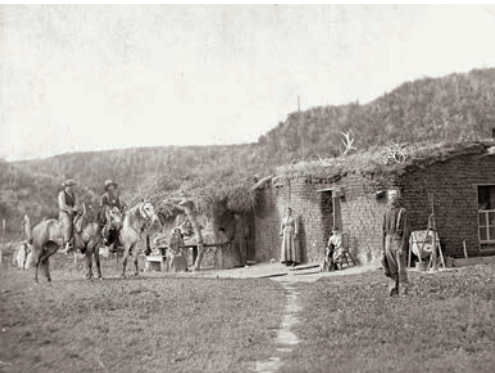
The Hartley family poses in front of their sod house on their ranch in Lillian Township on the Middle Loup River in Custer County, Nebraska, in 1886. Notice the antlers attached to the roof.
