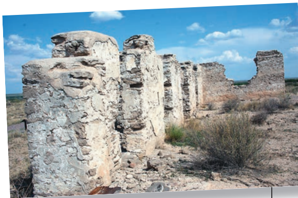
New Mexico's Fort Craig was established along El Camino Real de Tierra Adentro (the Royal Road to the Interior Lands), a Spanish Colonial trail that stretched 1,200 miles from Mexico City to Santa Fe.
