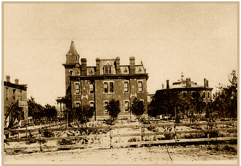
The Socorro County Courthouse and Jail were kept busy during Elfego Baca's terms as sheriff of Socorro County.
