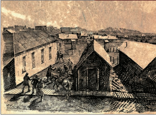
Backed into a narrow space.
