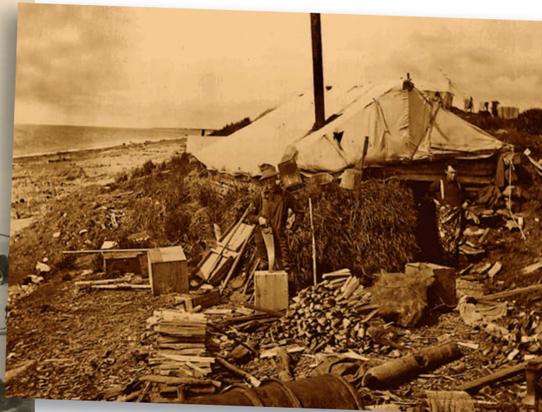
A miner's shack in Nome had sod insulation and driftwood for heat and a smokestack long enough (hopefully) to poke through the highest snowdrift.
