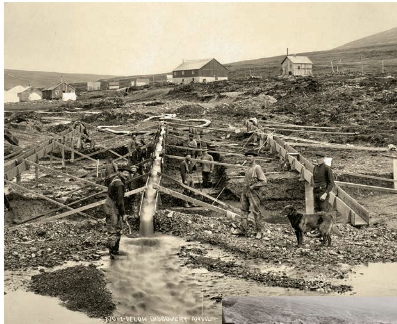
When the creek wasn't frozen over and covered in snow, miners sluiced gravel seeking their riches in gold along Anvil Creek near Nome, circa 1916.
