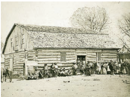
The first jail at Camp Supply or Fort Sill, circa 1868-74, was built of rough-cut lumber and timber with bars on the first-floor cell windows.
