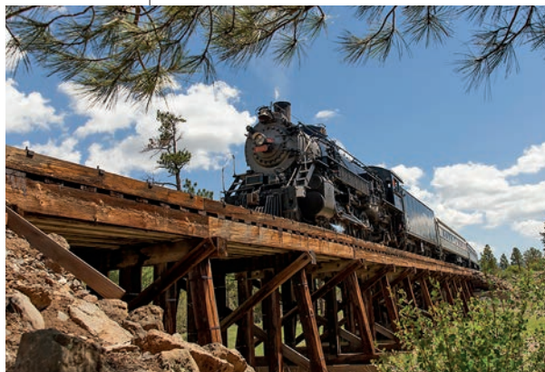
Grand Canyon Railway Williams, Arizona Courtesy Grand Canyon Railway
